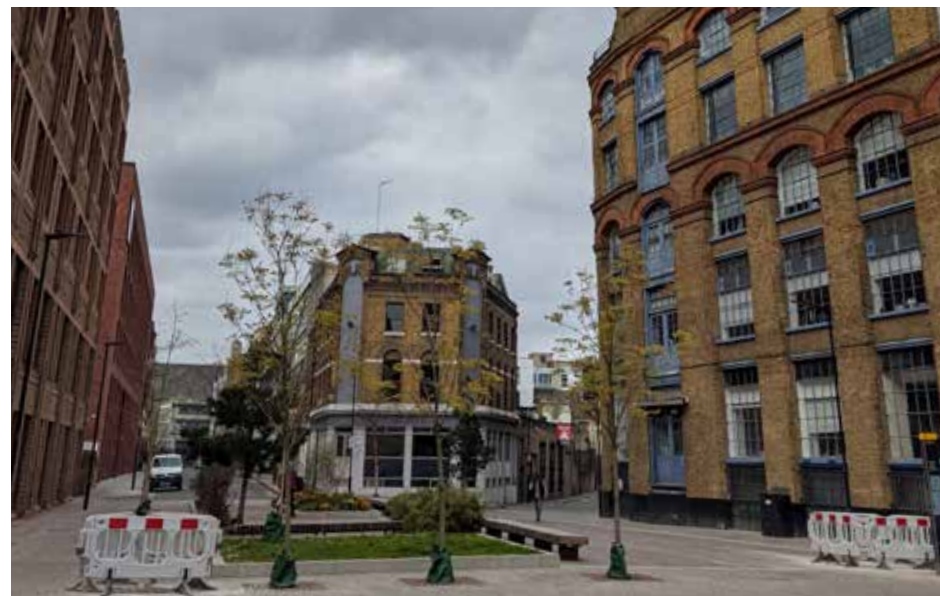
Public realm improvements at Worship Square
