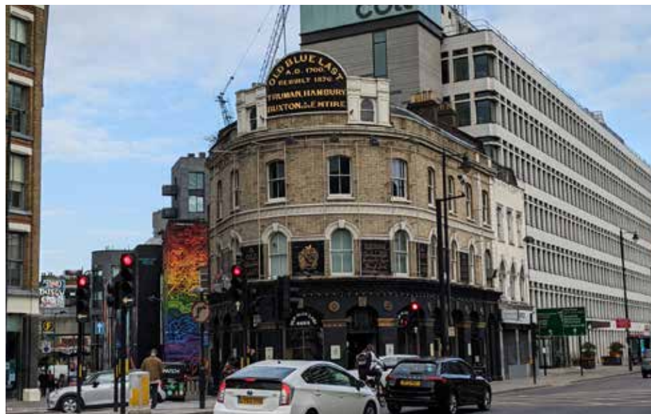
Old Blue Last, Great Eastern Street (Locally Listed)
