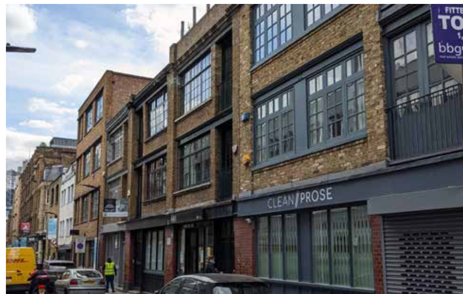
3 storey 19th century workshops on Charlotte Road
