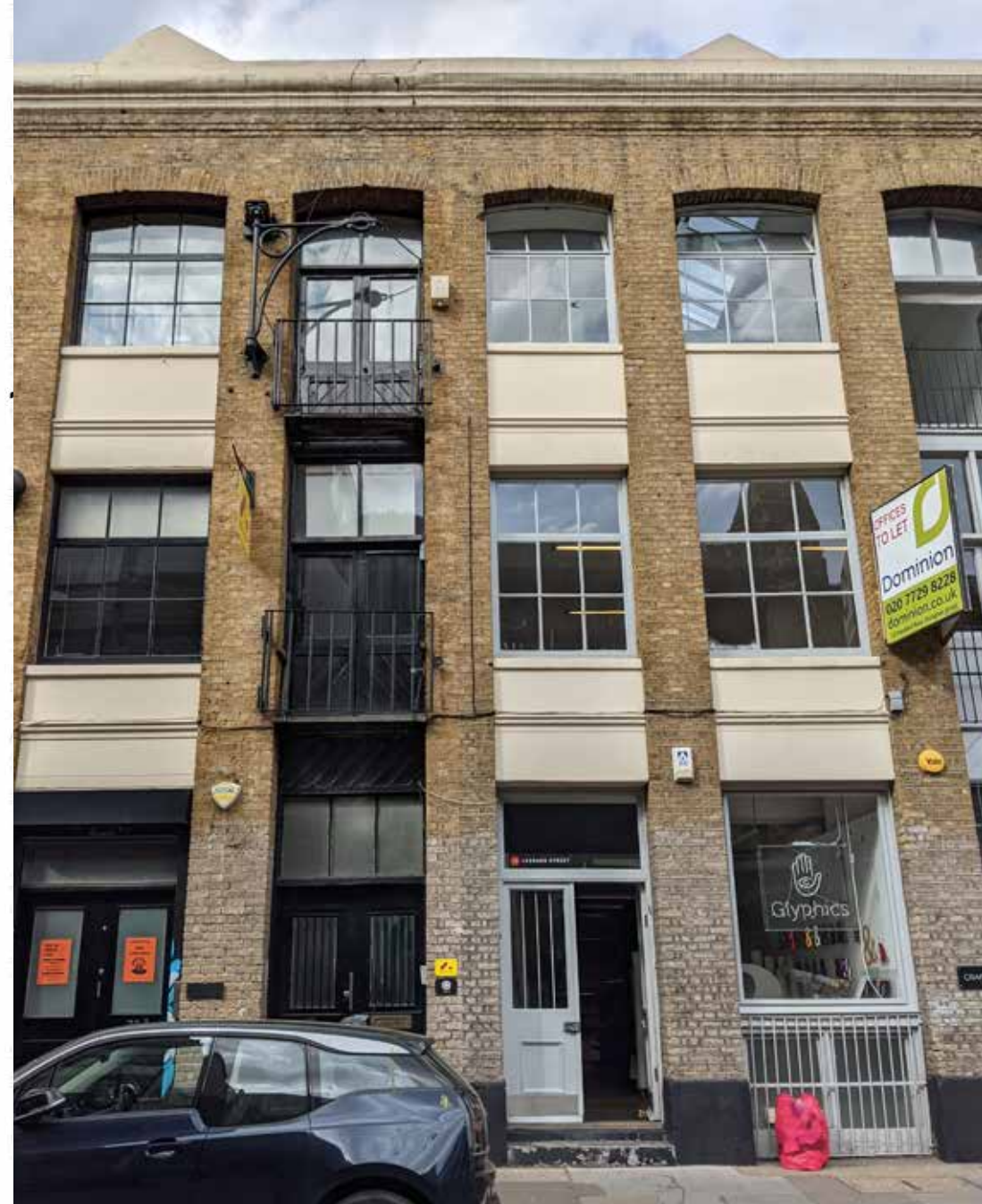
Leonard Street with typical Shoreditch details including deep reveals and vertical emphasis from windows and doors
