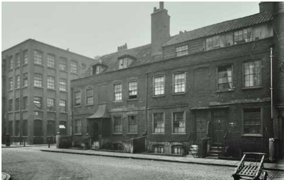
View south of Hoxton Square towards Rufus Street
