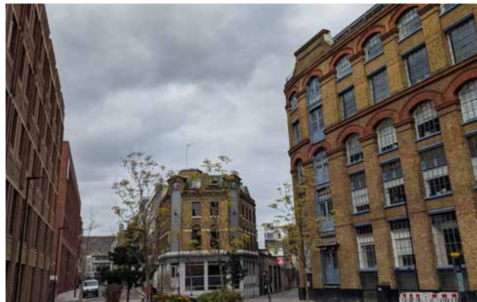
Clifton House, 75-77 Worship Street, Locally Listed
