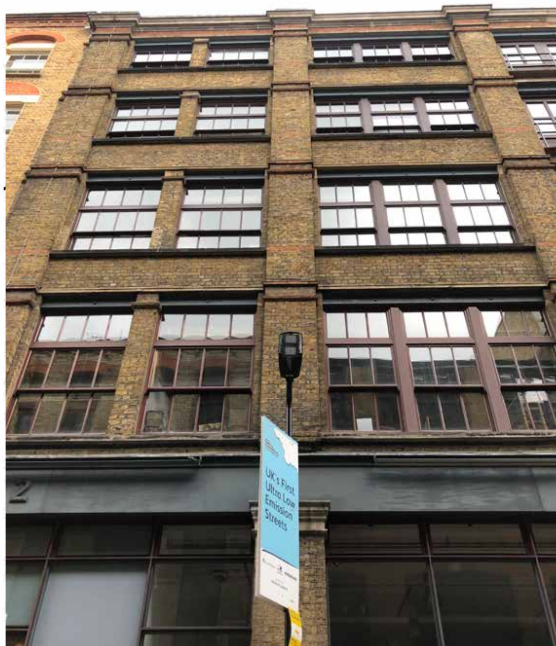
Charlotte Road with typical Shoreditch details including deep reveals and vertical emphasis from windows and doors
