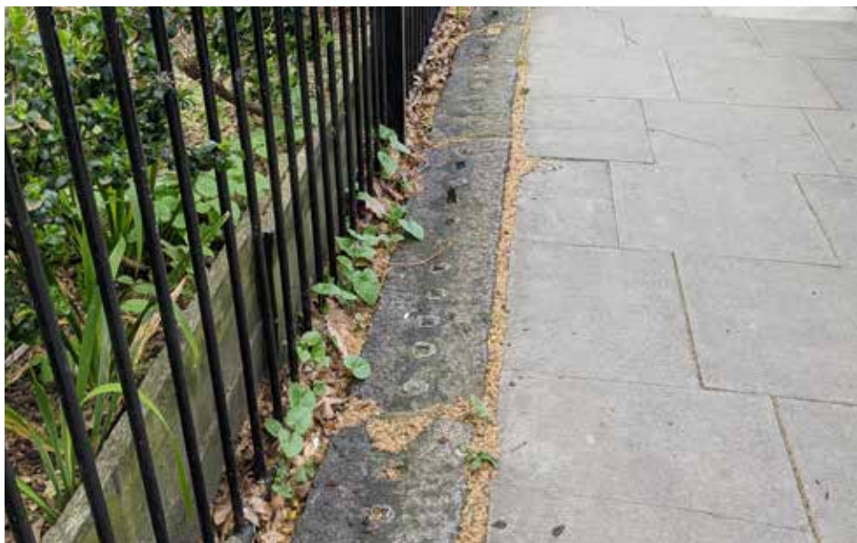
Modern railings with historic remains, Hoxton Square
