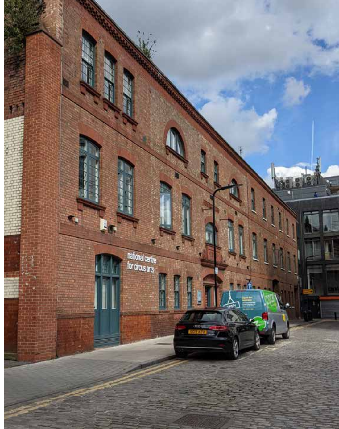
12 Coronet Street, former Electricity Power Station
