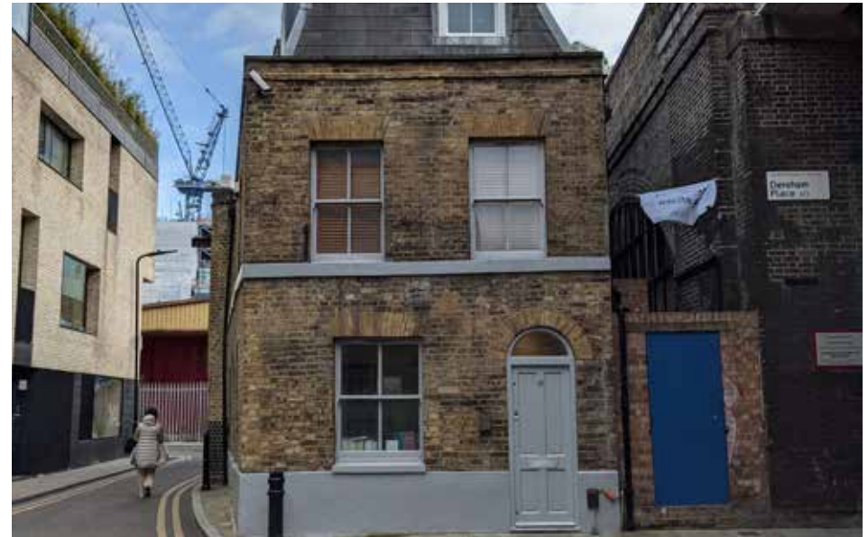
French Place: 2 storey property with later hipped mansard
